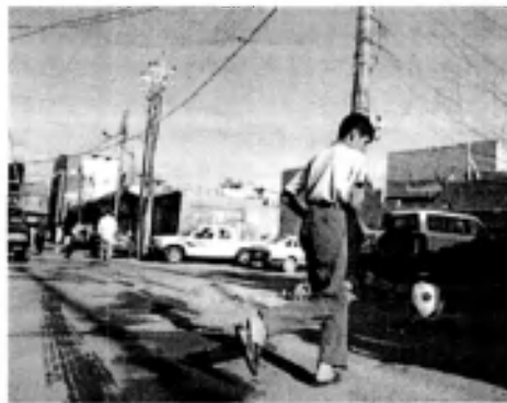
Wires from private generators over Erbil's back streets. (Karl Badohal)
