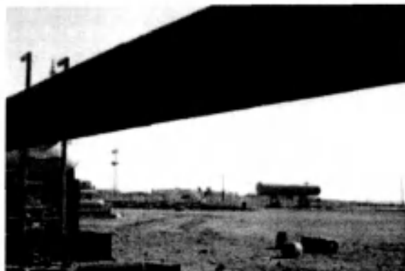
DNO's oil pipeline ends here at Faysh Khabur, near the Iraq border with Turkey and Syria. It's less than a half mile from the Iraqi government's oil metering station, seen in the background, but a deal hasn't been reached between Baghdad and the Kurdistan Regional Government to allow exports from KRG inked deals. (Ben Lando/UPI)
