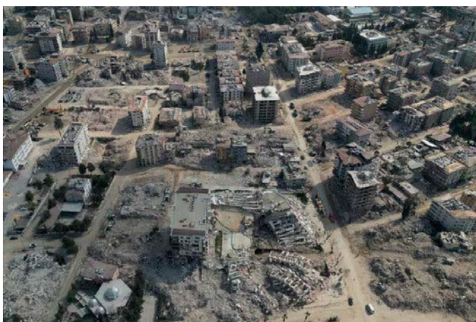
The collapsed Guclu Bahce complex in Antakya, Turkey, in March. Sergey Ponomarev for The New York Times
