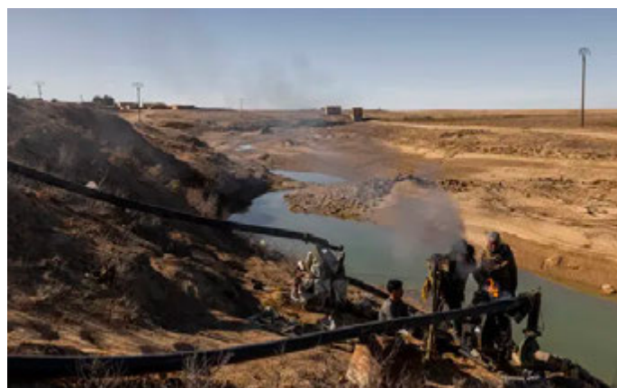
Irrigation pumps on the Khabur River, which has slowed to a trickle. Now the pumps have to work overtime, using more diesel fuel to get the same amount of water. Credit...Ivor Prickett for The New York Times
