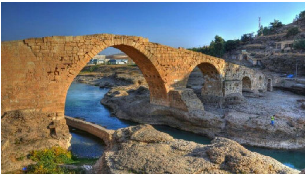
Zakho's historic Delal Bridge. (Photo: Goran Sabah Ghafour/K24)
