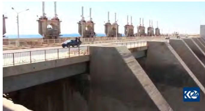
The Tabqa dam provides most of the electricity to the northeast (Photo: Kurdistan 24).
