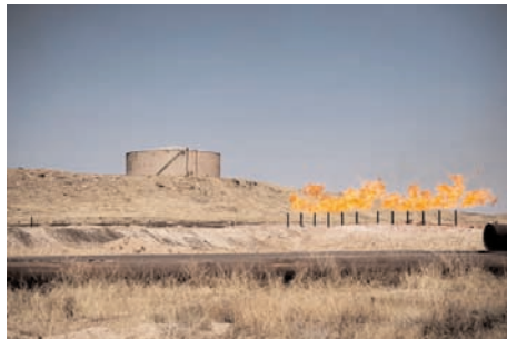
Gas burn-off and oil tanks at the northern oil fields in Kirkuk, Iraq. Kurdish officials angered Baghdad by exporting oil produced in their region directly to Turkey. Credit Andrea Bruce for The New York Times
