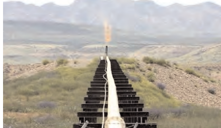
A flame rises from a pipeline at Tawke oil field. The Kurds have begun to export oil to Turkey through a new pipeline independently in direct defiance of Baghdad. Azad Lashkari / Reuters
